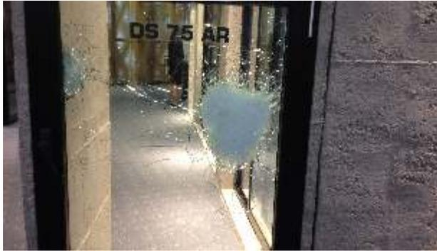
Counterattack glasses are the laminated combination with main layers of PVB, polyurethane and polycarbonate. The glass plates can be used as tempered glasses when necessary. The total resistance of those glasses are closely related to the properties of the carrier. The counterattack units consist of three categories as the ones resistant to impact, the ones resistant to undesirable passes and robbery and the ones resistant to firearms.
