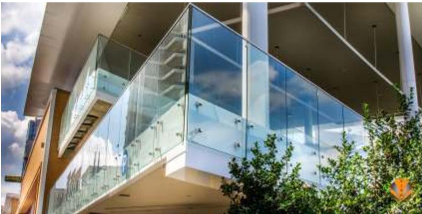
The structures needing to use safety glasses are indicated in the "TSE 13433 Glasses – Used in the Structures – Codes of Practices for Safety Related to Human Crash". As indicated under this standard, those glasses should be especially used for the places where the glass-shattering has dangerous consequences.
